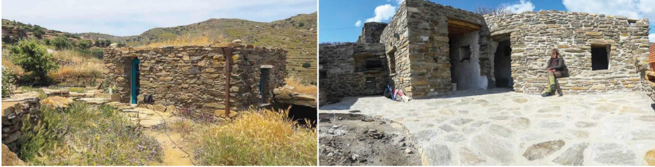
Figure 4.12 Final state of renovation of the stables
