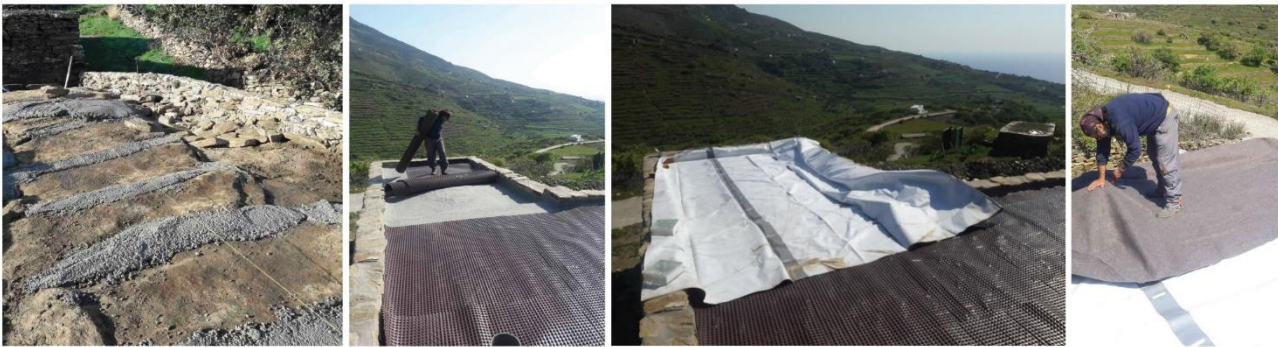
Figure 4.9 Construction of stable roof
