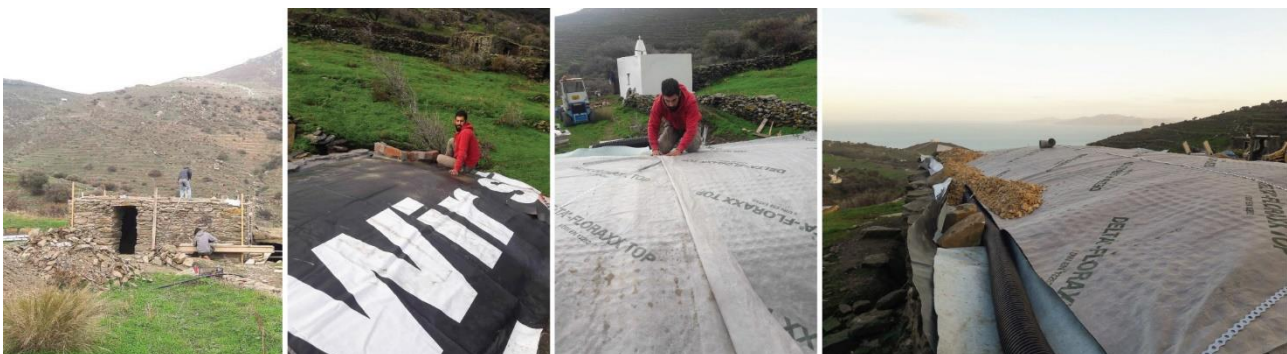
Figure 4.10 Installation of the upcycled PVC membrane
