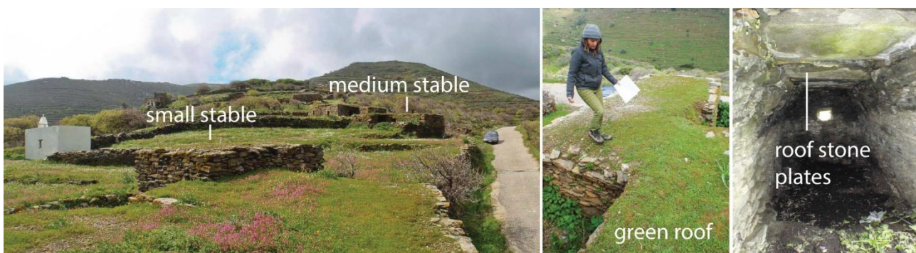
Figure 4.5 Picture of the stables, green roof and roof stone plates
