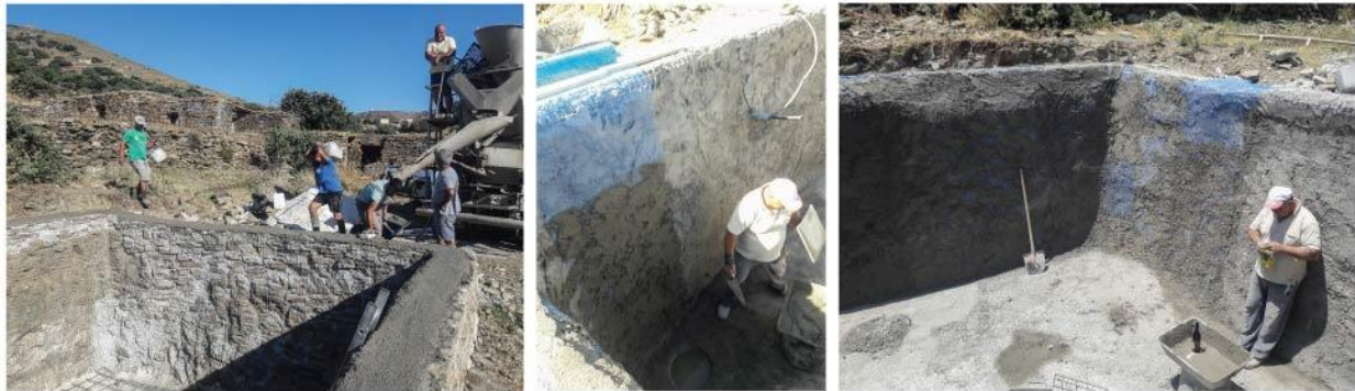
Figure 4.4 Plastering process
