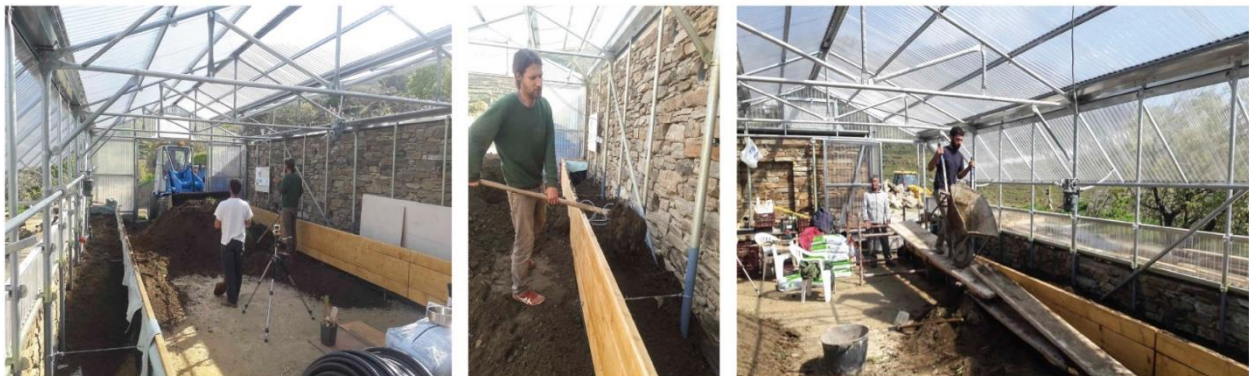
Figure 5.5 Construction of the greenhouse interior
